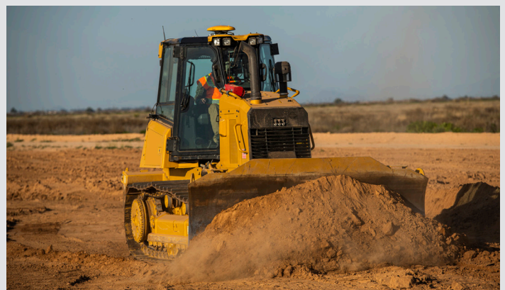
SITE PREPARATION - COARSE GRADING
